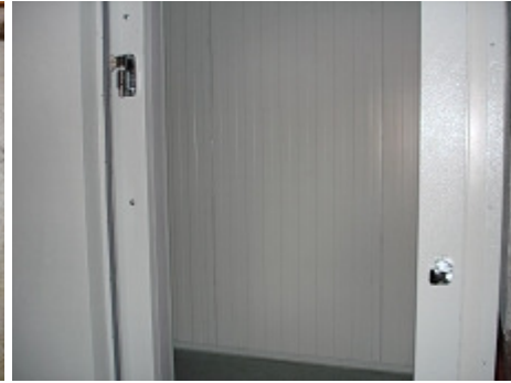
Interior of new freezer
